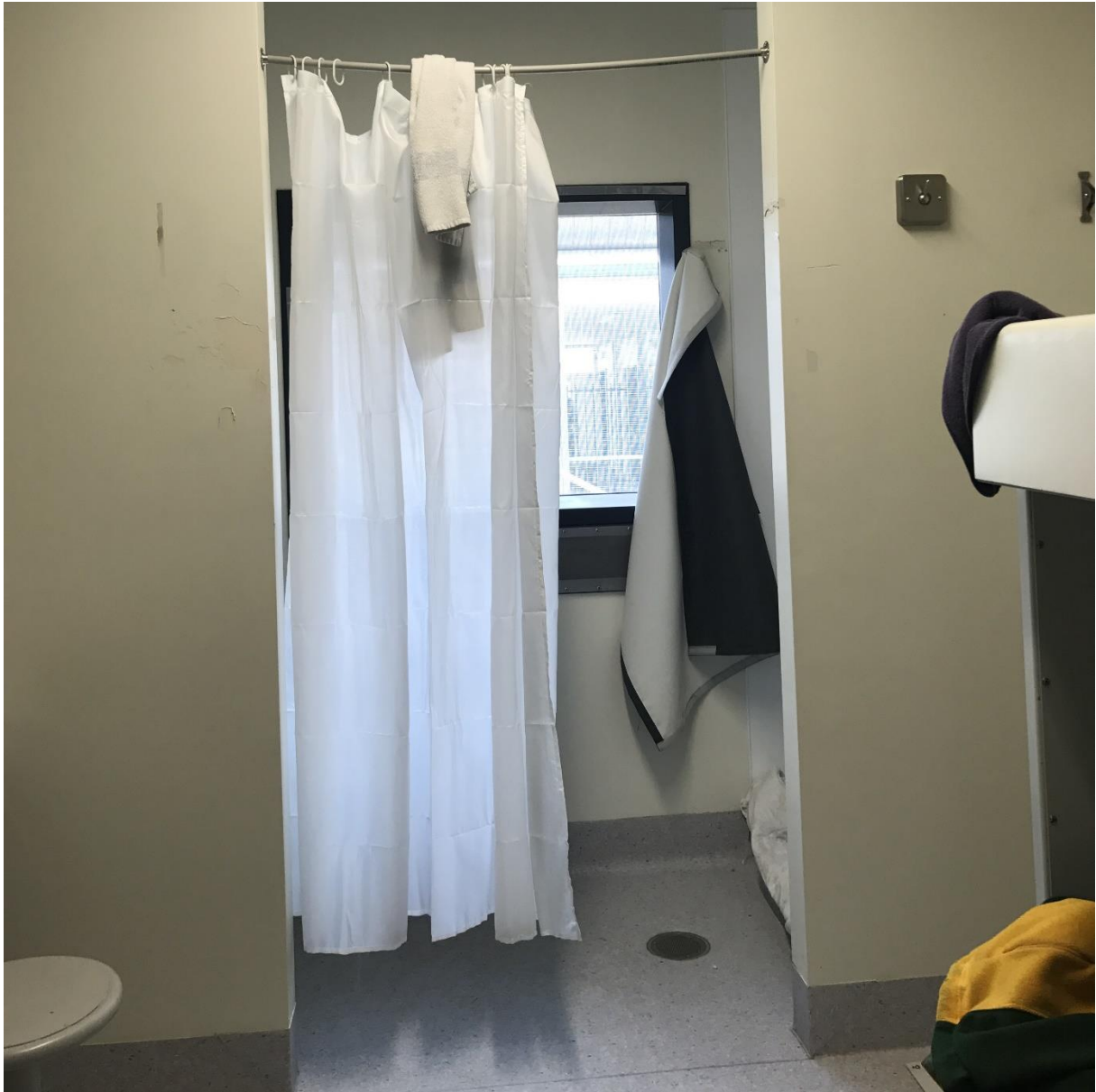
Curtain separating bathroom from sleeping quarters, Fraser compound, BITA
