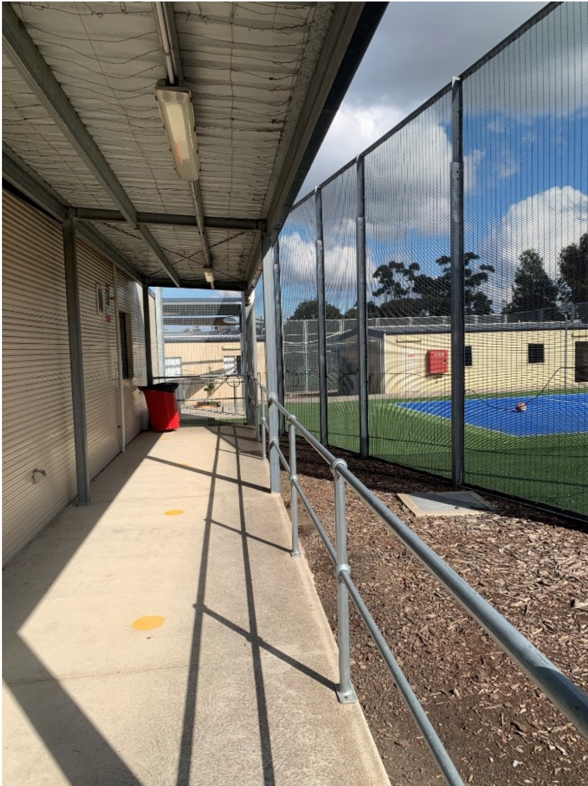
Photo 20: Fenceline separating canteen window from Bass 1 outdoor area (MIDC)
