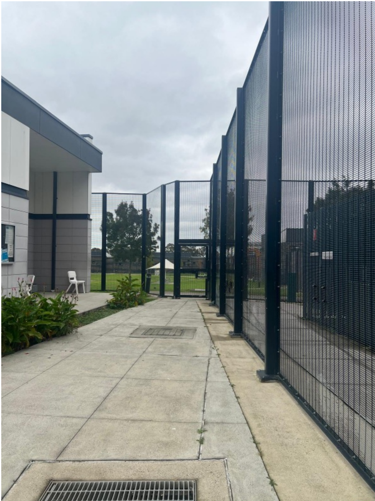
Photo 25: Fencelines separating Cowan compound from Lachlan compound (right) and Community green (ahead) (VIDC)
