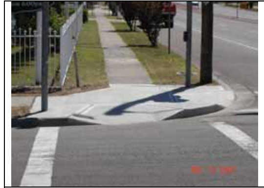
Dishramps at Adelaide St. and Glenelg St. Raymond Terrace
