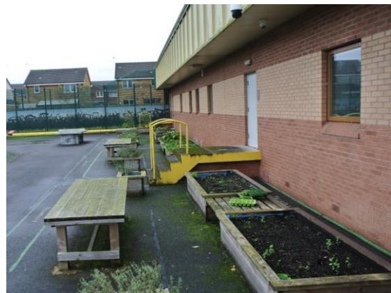
186. Kibble Safe Centre, Rear yard, planter beds
