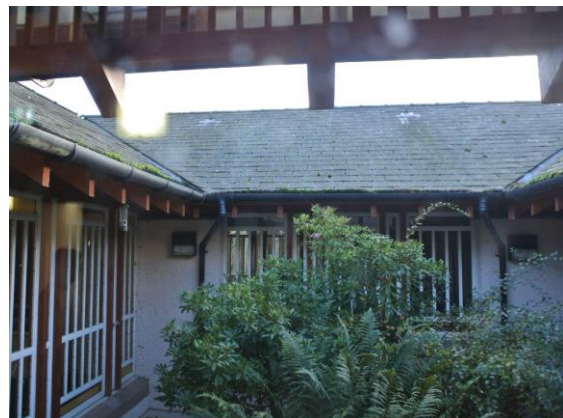
203. Rossie, School building, lightwell
