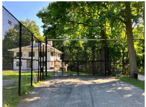
27. Crest House LSP, Perimeter fence
