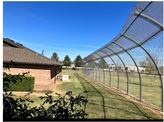
93. Mt Vernon, Perimeter fence
