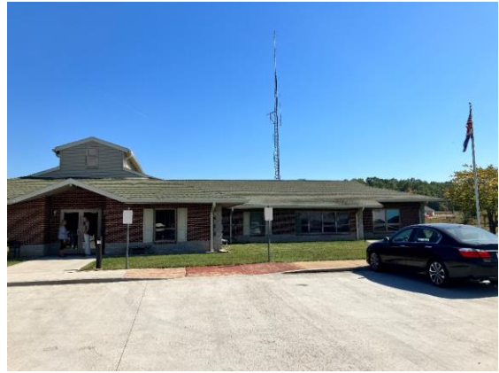
125. Gentry Residential Centre, Cabool MO, 2022
