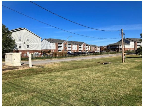
69. Excel Centre, Context
