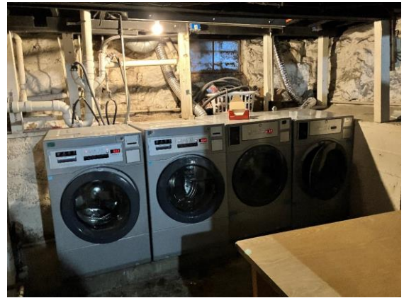
77. Datema House, Basement laundry
