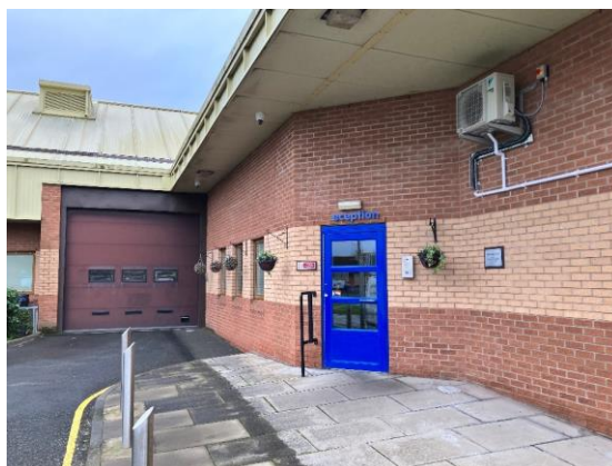
176. Kibble Safe Centre, Entry
